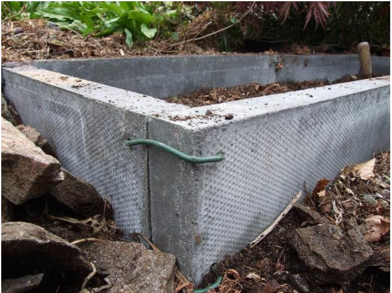
Joining corners
